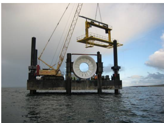
Towing jack-up barge 'Octopus' to installation site.
